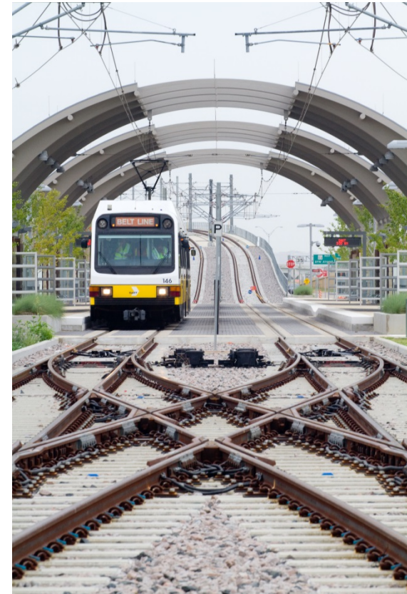
A crossover connects two parallel rail tracks, allowing a train on one track to cross over to the other.
