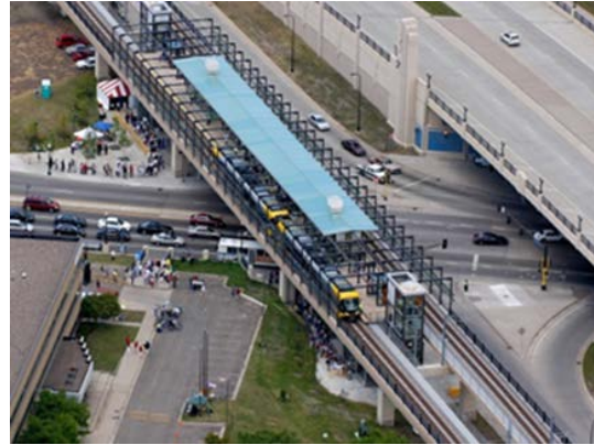
Typical Aerial Station
