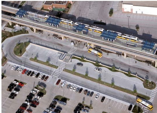
Typical Park-and-Ride Station
