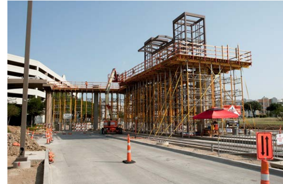
Light rail station construction traffic control
