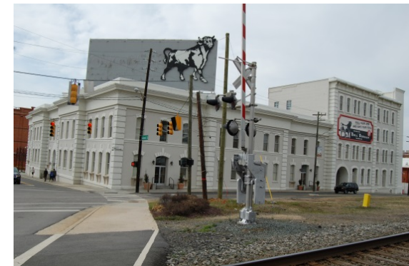
American Tobacco Company Manufacturing Plant
