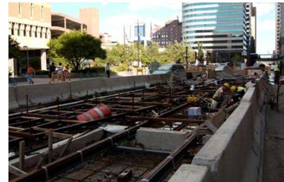
Example of Embedded Track Construction
