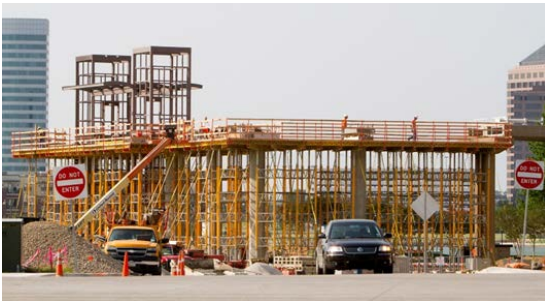
Light rail station construction of roadway crossing
