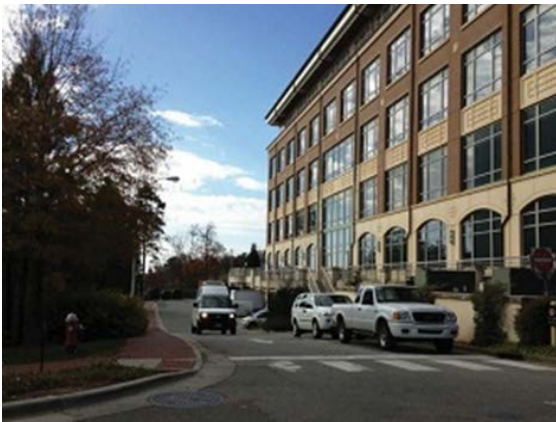
UNC Medical Facility
