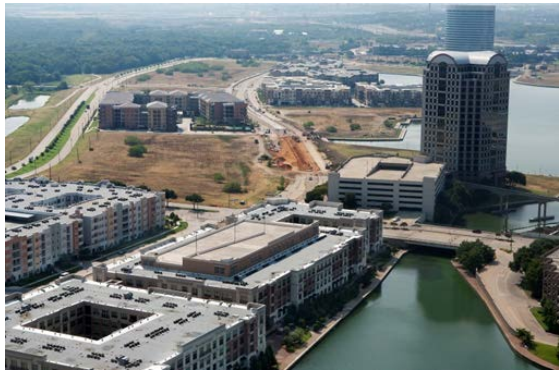
Light rail construction in business center
