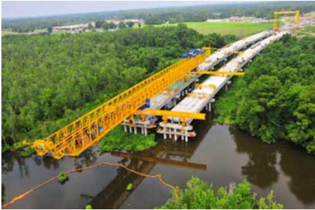
Example of Top Down Bridge Construction in Sensitive Natural Areas
