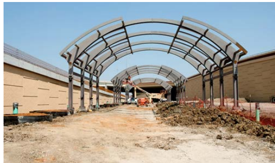
Light rail station construction BMPs to contain stormwater runoff
