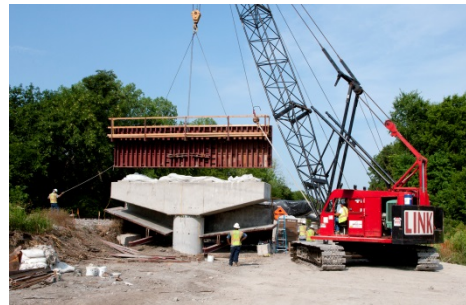
Example of Light Rail on Elevated Structure
