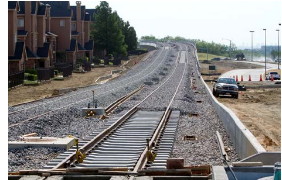
Light rail construction near neighborhood
