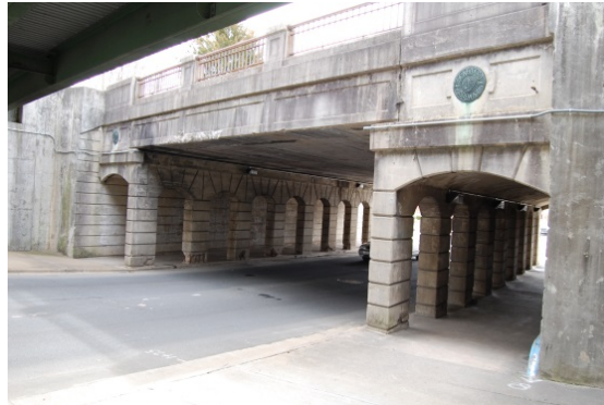
Southern Railway Bridge
