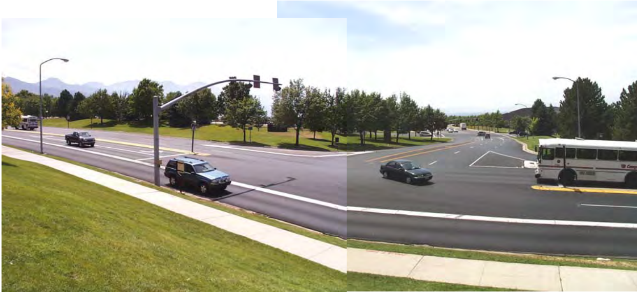
South Campus Drive/Campus Center Drive Intersection before the Roundabout Construction. Yield signs control the traffic along the top of the T-intersection. Bypass lanes existed at the two corners and across the top of the “T”. Because of the existing free movements the change to a roundabout operation was not as extreme for drivers.
