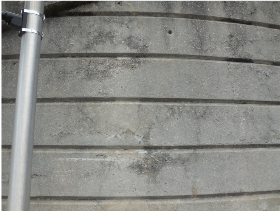
Figure 1-2 Map cracking on southwest wing wall
