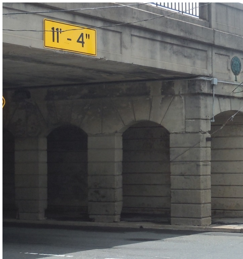
Figure 1-1 Spalls at base of columns and vehicle impact damage to fascia beam
