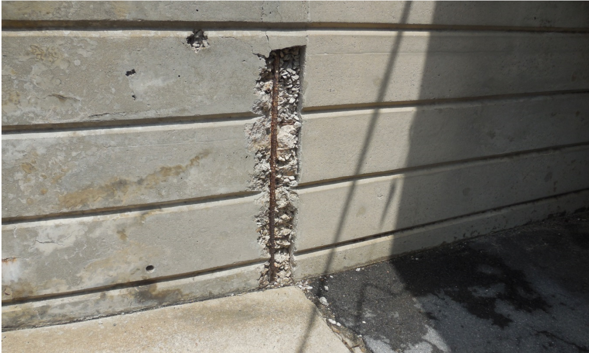
Figure 1-3 Spall at abutment joint with southwest wing wall
