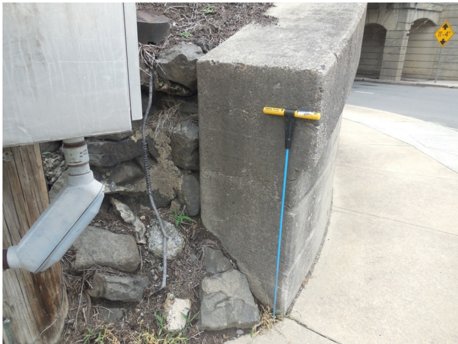
Figure 1-4 Probe used to estimate spread footing depth
