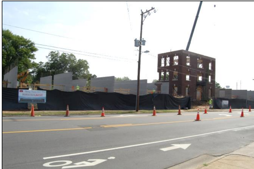
Figure 141: Former McPherson Hospital Main Building in September 2014 during construction of Marriott hotel
