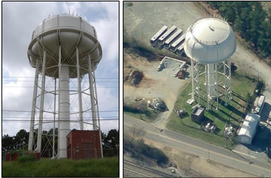
Figure 219: Durham Water Tower and Valve House: looking south
