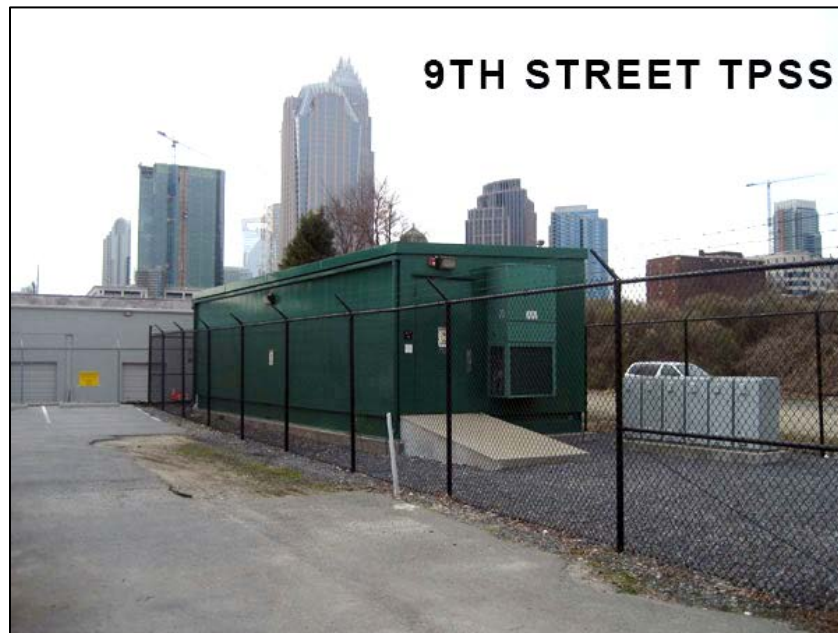
Figure 10: Traction Power Substation in Charlotte, North Carolina (source: charmeck.org/city/charlotte/cats/planning/ArtinTransit/inprogress/Pages/BLE-TPSS,SH,CCs.aspx )
