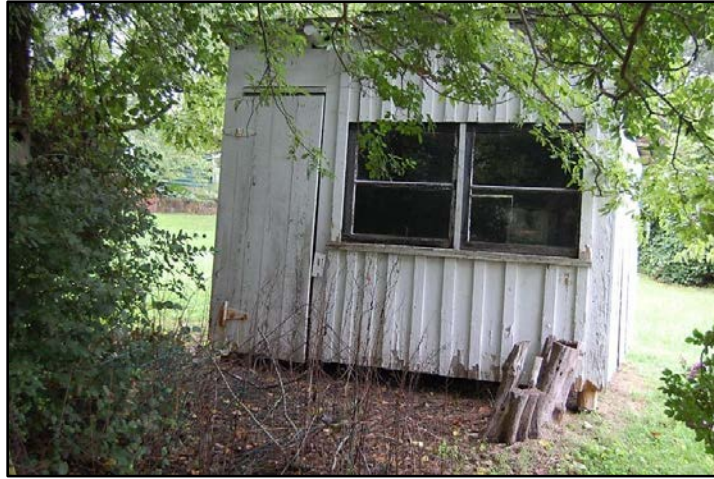
Figure 90: Playhouse [F]: east rear and south side elevations (c1935 – contributing)
