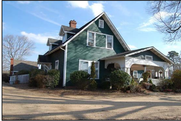
Figure 87: Milkhouse/Washhouse [B]: south gable and east side elevation (c1918 – contributing)
