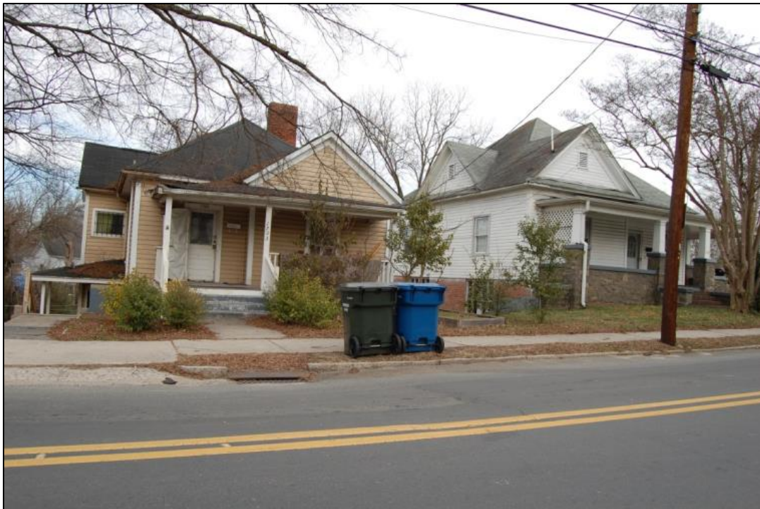
Figure 223: East Durham Historic District: south facades of 1703 and 1705 Angier Avenue, left to right
