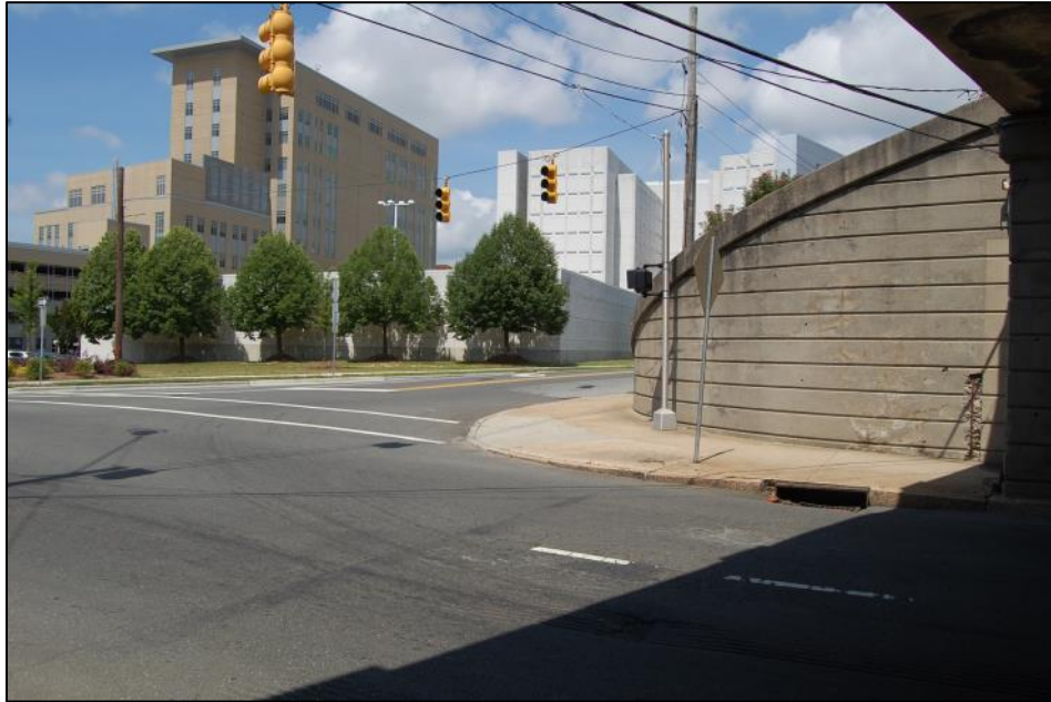
Figure 201: View looking south west from bridge at intersection of East Pettigrew Street and South Roxboro Street toward Durham County courts building at left and jail at center; proposed project would run in near lane of Pettigrew Street
