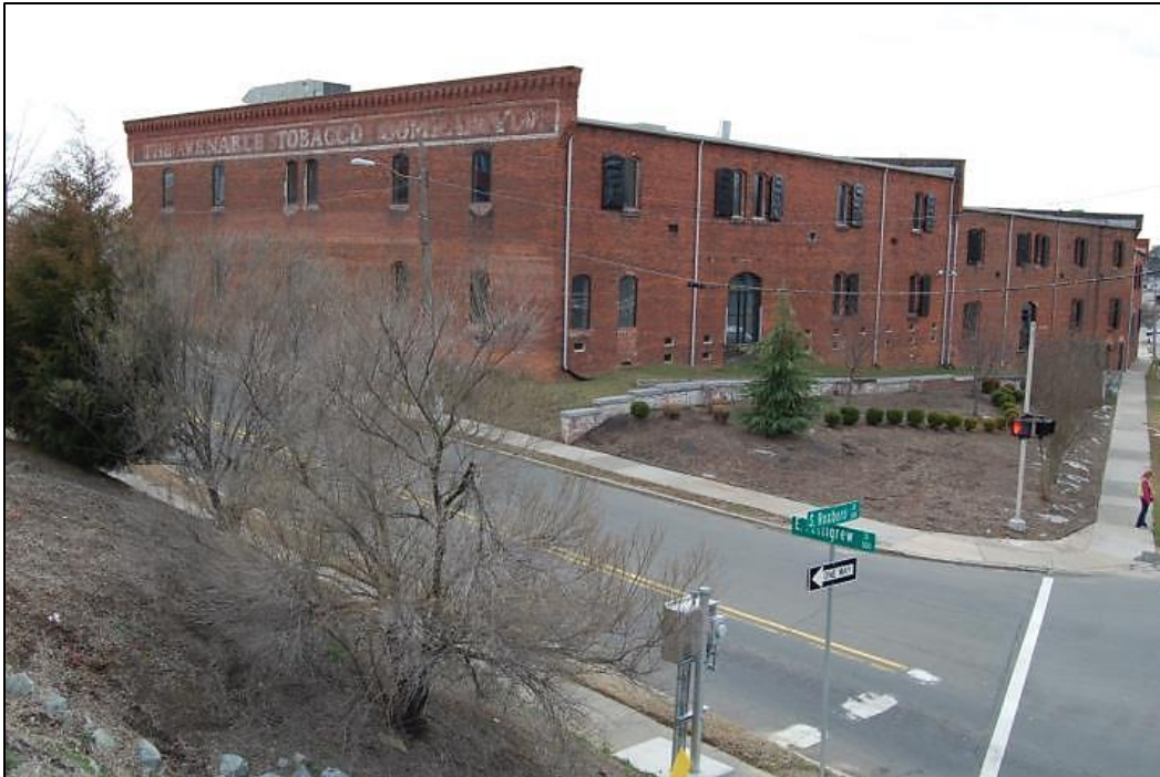
Figure 202: Venable Tobacco Company Warehouse: north and west elevations from elevated railroad alignment
