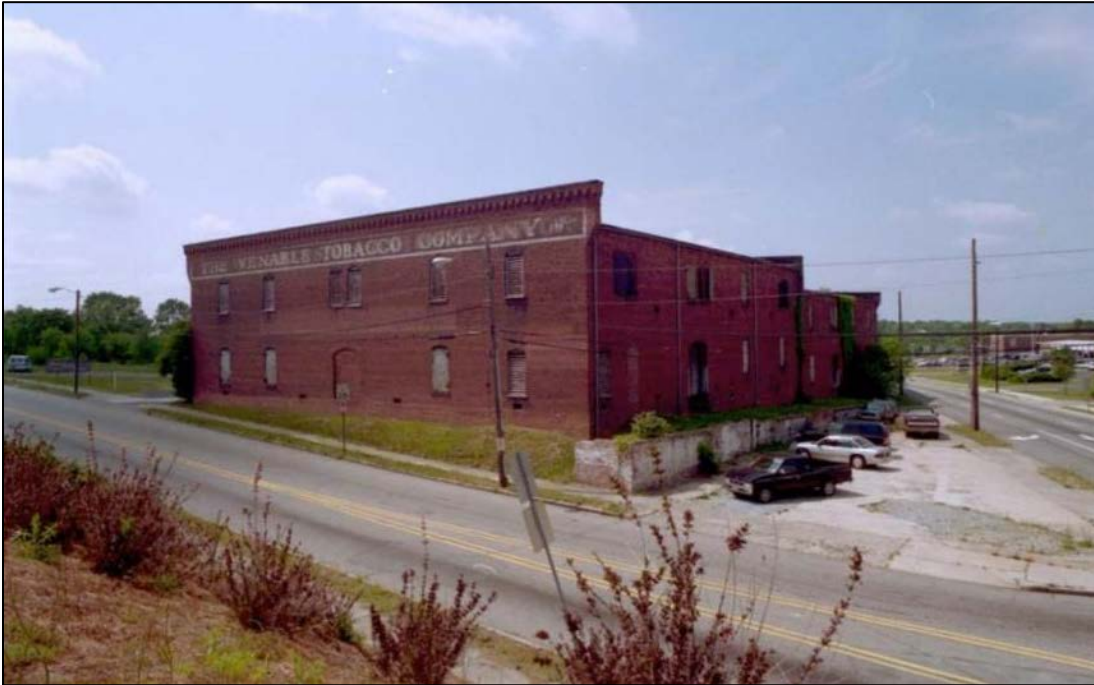
Figure 213: Looking southeast from tracks at warehouse across Pettigrew Street; note that separate triangular lot that held filling station is vacant, 1989 (source: http://www.opendurham.org/buildings/venable-tobacco-company and Durham Herald Sun )
