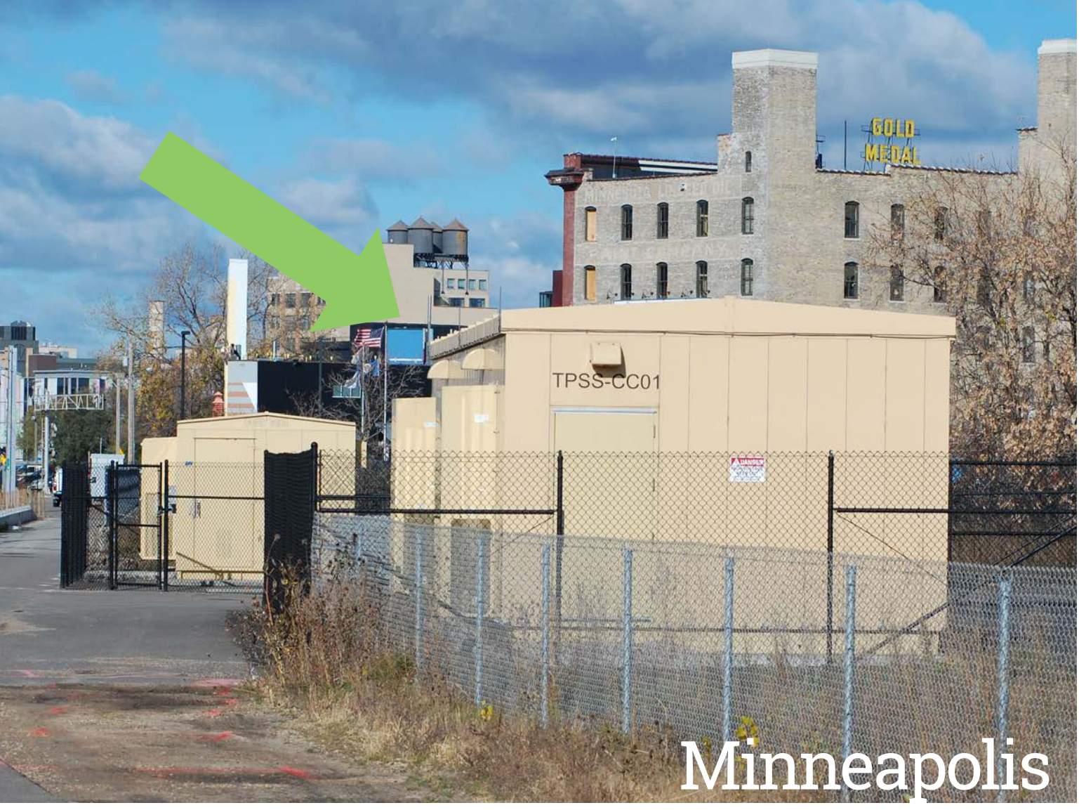
Traction Power Substation
