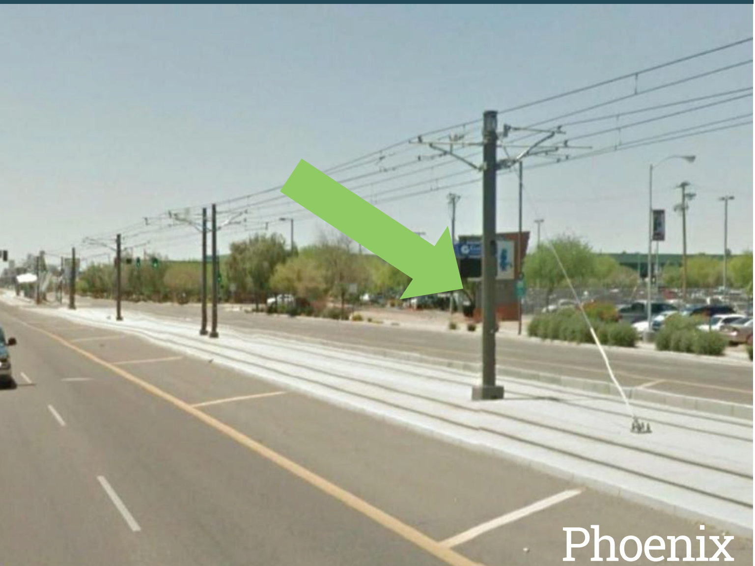
Overhead Catenary System - Poles
