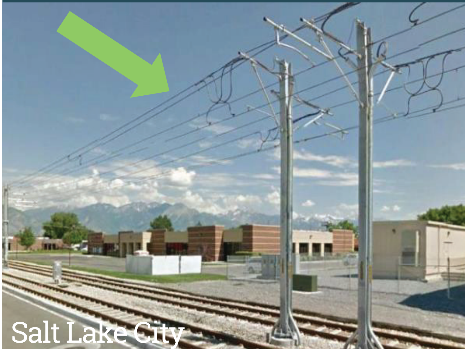
Overhead Catenary System - Wires
