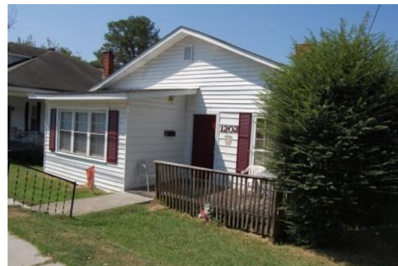
1202 S Alston Ave [1920s] (photo above)
