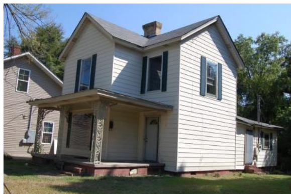
911 S Alston Ave [1910s] (photo above)
