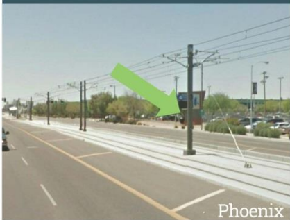
Overhead Catenary System - Poles
