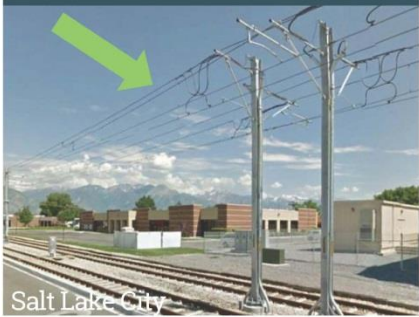
Overhead Catenary System - Wires
