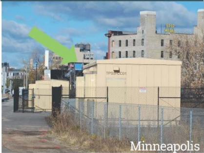
Traction Power Substation
