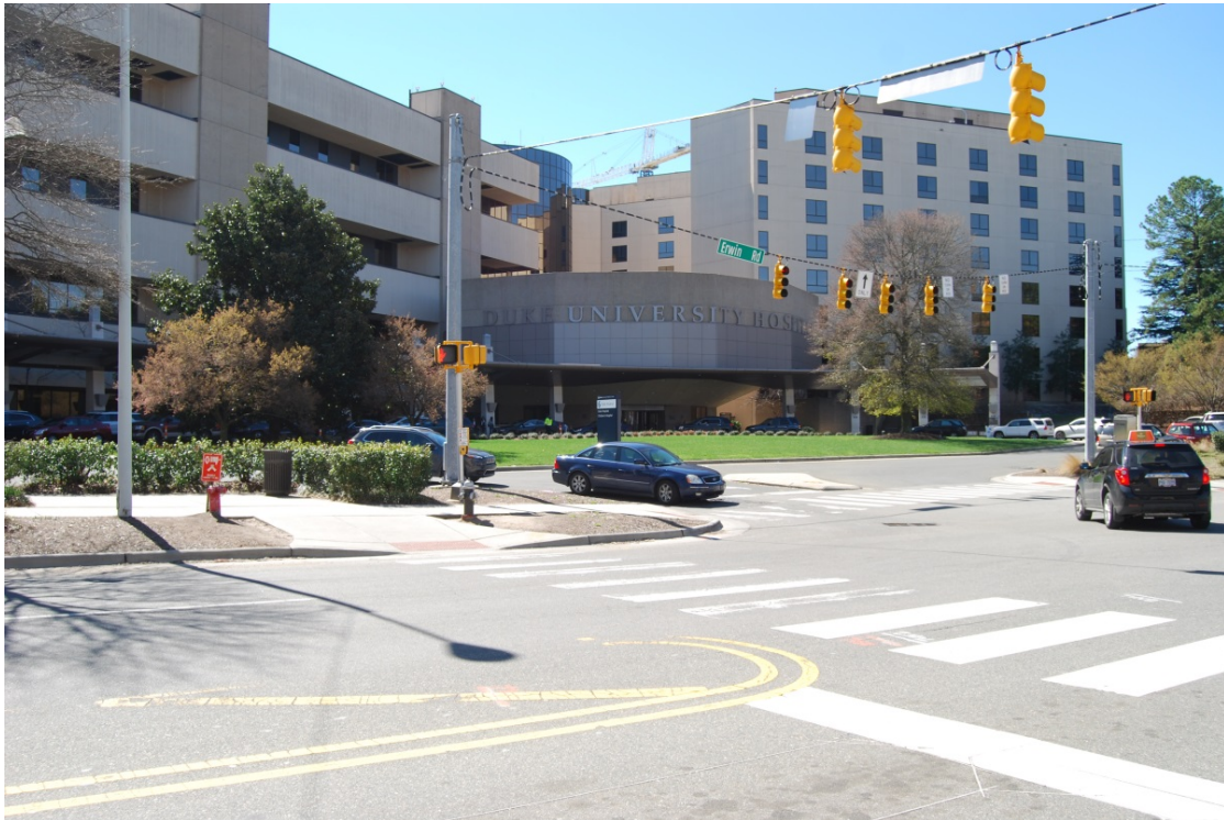
Figure 5-14: Erwin Road (Facing South across the Median; Location near the Proposed Elevated Duke/VA Medical Centers Station)
