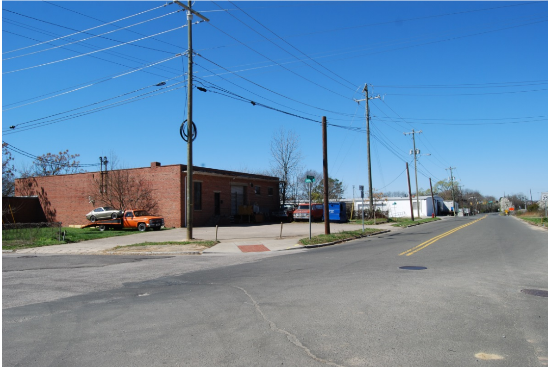
Figure 5-22: Pettigrew Street (Facing Northwest from near Alston Avenue)
