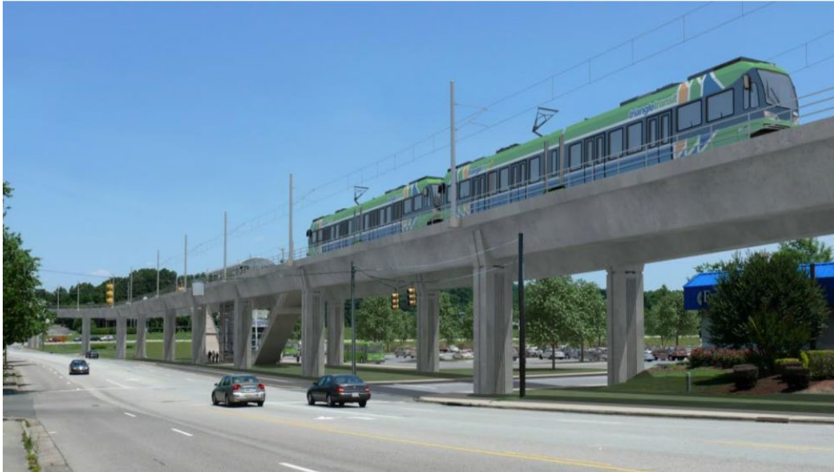
Figure 5-15: Typical Elevated Section
