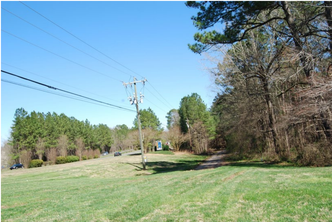
Figure 5-4: Downing Creek Parkway and Stancell Drive Intersection (Facing Northeast; Location of Proposed Elevated Section at NC 54)
