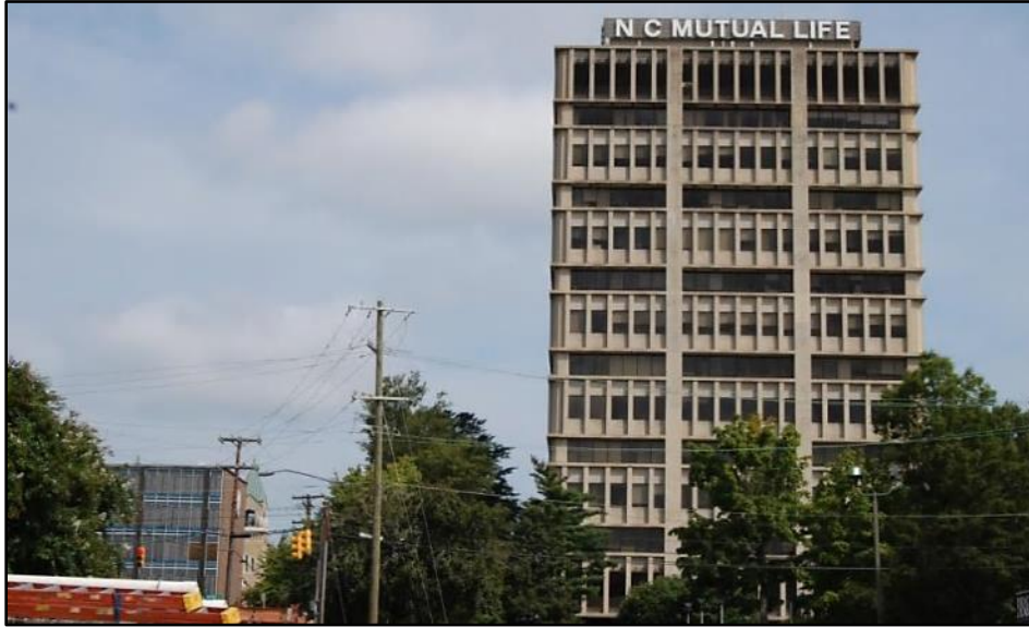
Figure 4-25. North Carolina Mutual Building (DH 2477)
