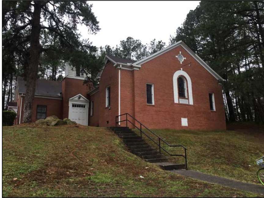
Figure 4-1. Asbury Temple United Methodist Church (DH 3964), view looking west from E. Lawson Street.
