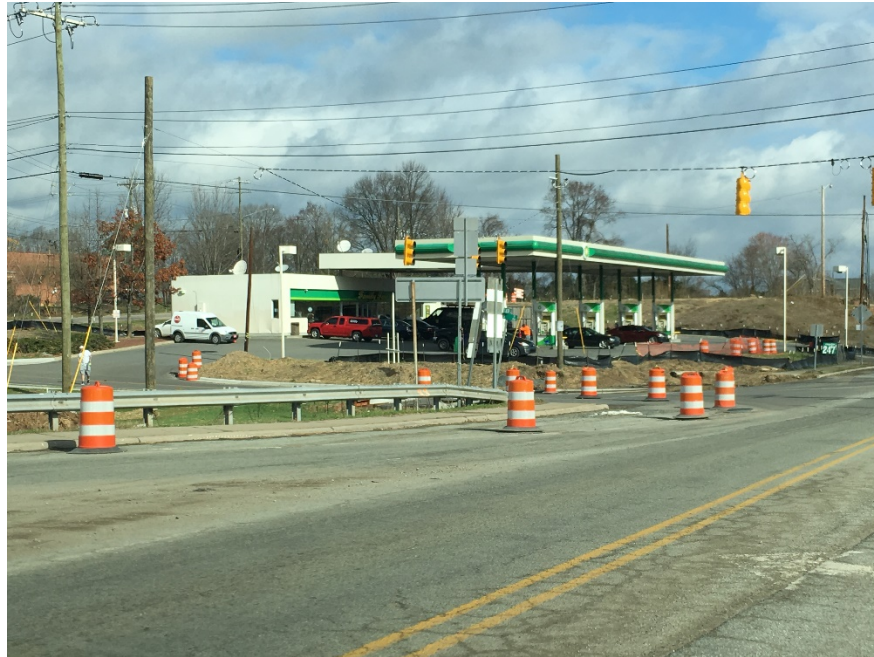
Photo 9: Existing freeway BP Station located near intersection of Pettigrew Street and Alston Avenue (ongoing UST, LUST, LUST TRUST regulatory listings). View is to the north.
