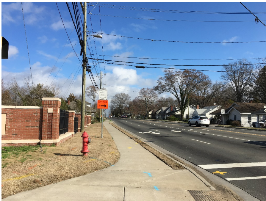
Photo 10: Future location of NCCU Station (near NCCU residence LUST). View is to the north.
