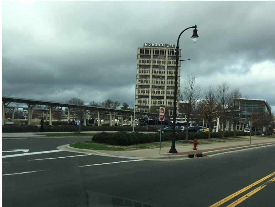
Photo 7: Future LRT Project Durham Station (expansion of existing bus station). View is to the northwest along West Pettigrew Road.
