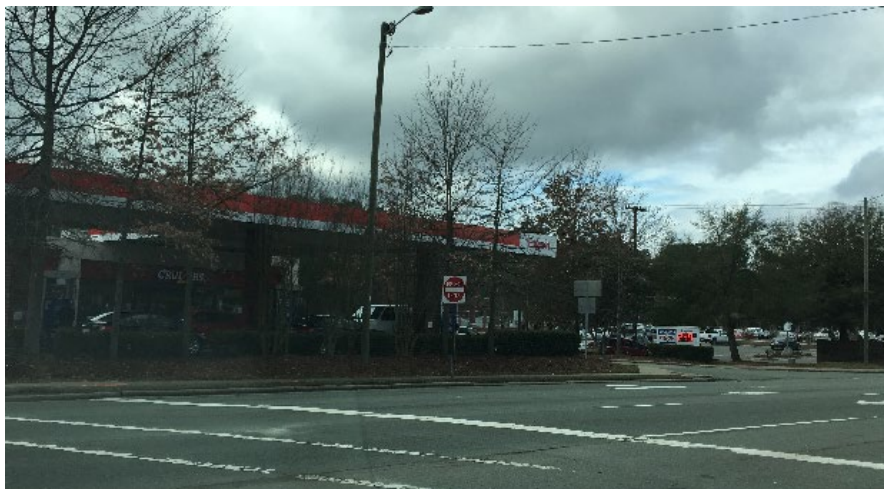
Photo 2: Current Exxon Station (previously identified as a LUST Medium and elevated to high, with increased proximity to the corridor). View is to the west.
