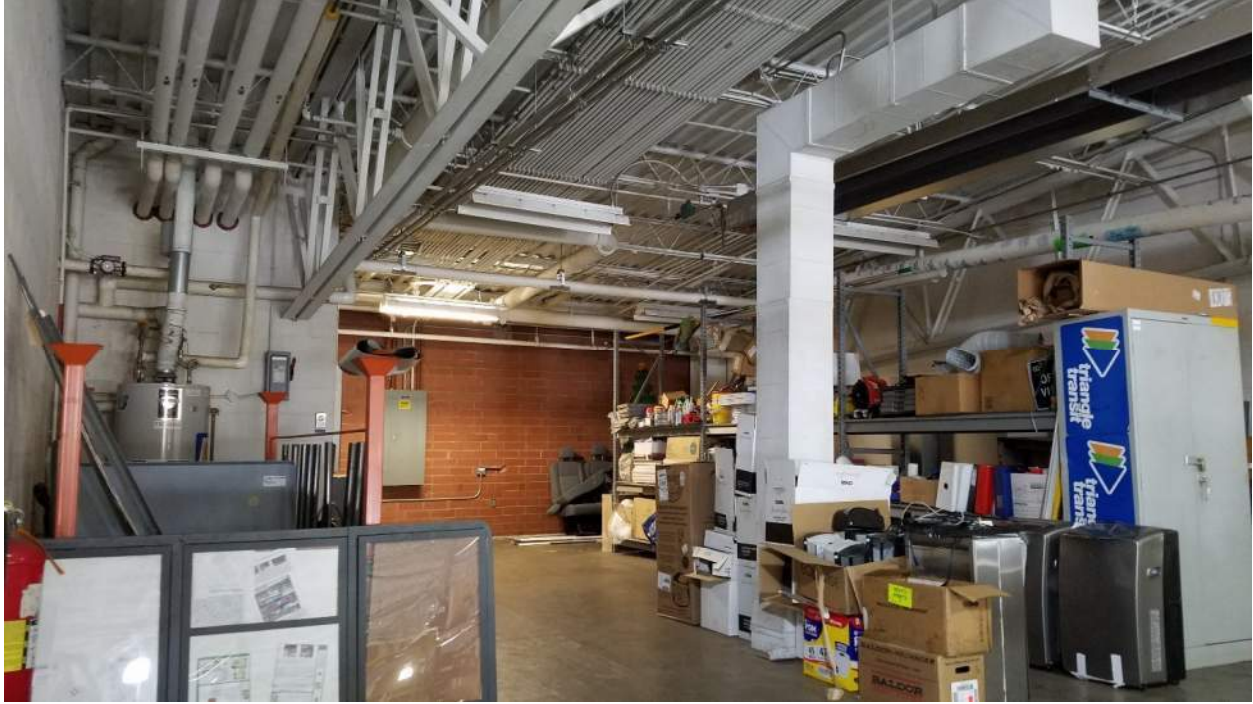
Mezzanine West Side
